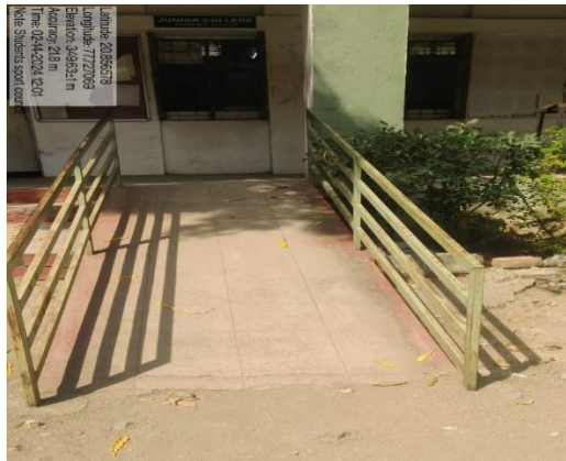
Ramp at Office
