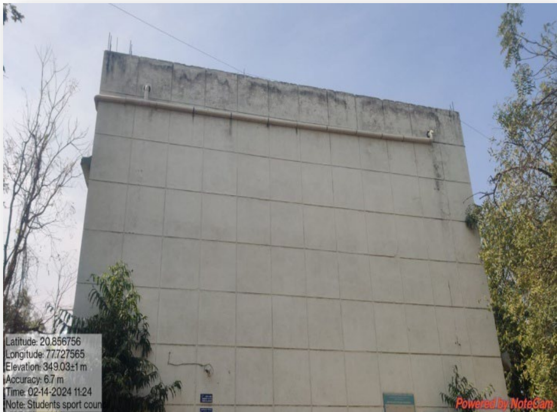
Rain Water Harvesting Plant
